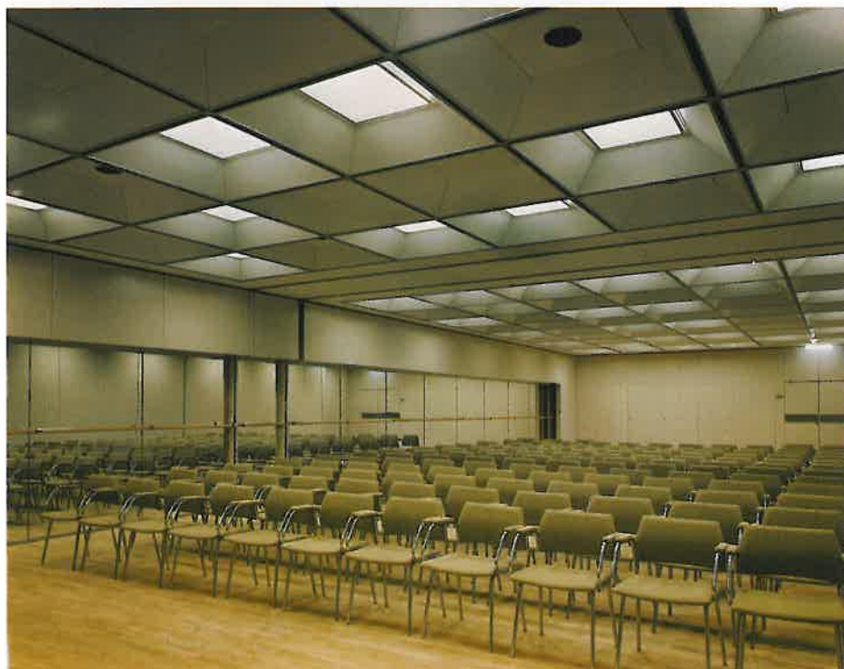
Two committee rooms. A virtue has been made of the uneven flashing of the leaf-lite ceiling, due to limited head-room, as it relieves the monotony of the ceiling. In the room shown below a Programme 2 ceiling has been installed.
